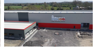
Patterson Pump Ireland
