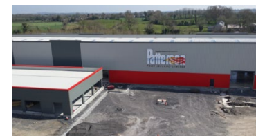
Patterson Pump Ireland
